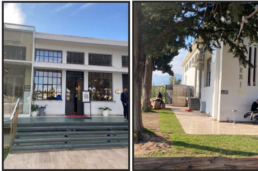
Figure 15. Entrance and disabled lift of Cemil Meriç library in Dokumapark
