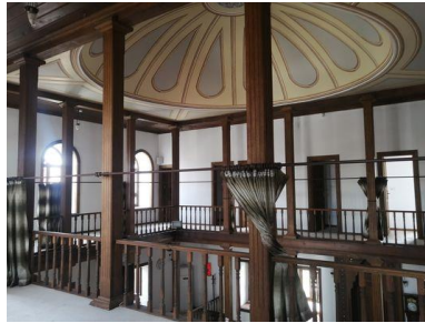
Figure 17. Balcony level gallery void (Demirkol, Burçin İrem Demirkol Photo Archive, 2023)
