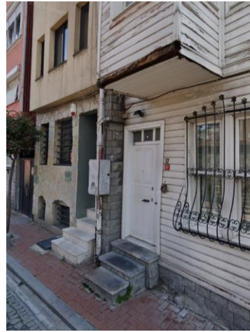
Figure 11. Building entrances in Arnavutköy Dere Street (Google Maps)
