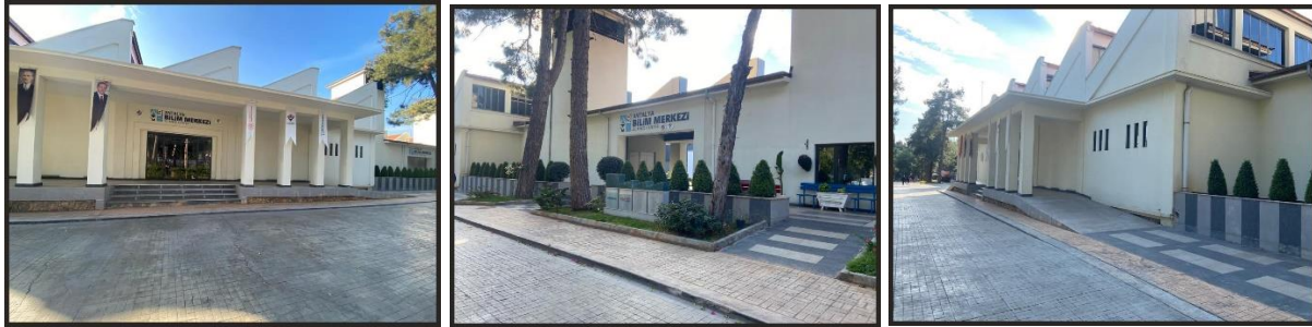
Figure 17. Entrance, ramp and stairs of Antalya Science Center in Dokumapark
