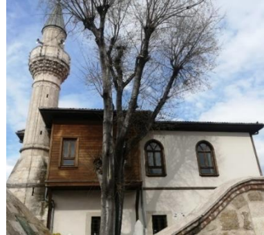
Figure 12. Mosque northeast facade
