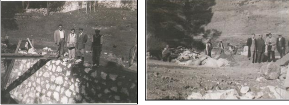
Figure 9. The water tank construction works in the Bursa Mevlevîhâne garden, 1953 (Elbas & Alkan, 2023, 37)
