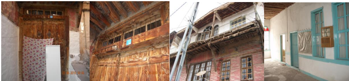
Figure 15. The ground floor features a double-winged wooden sentence door of the building, wooden handrails supporting the protrusion on the south facade, and the upper floor's inner living area with rooms (Sille Street Rehabilitation Survey Report, 2014).
