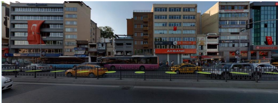
Figure 22. High-storey reinforced concrete buildings on the Beşiktaş Street (Google Maps)
