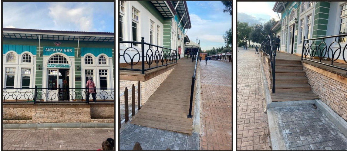
Figure 24. Entrance, ramp and stairs of train library in Dokumapark
