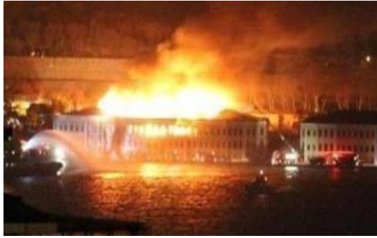
Figure 3. Galatasaray University burned down on 22 January 2013 due to a short circuit in the electrical installation (Source: www.yesilgazete.org )
