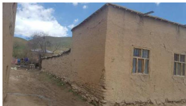
Figure 8: Başkale rural houses built with adobe, stone and wood materials
