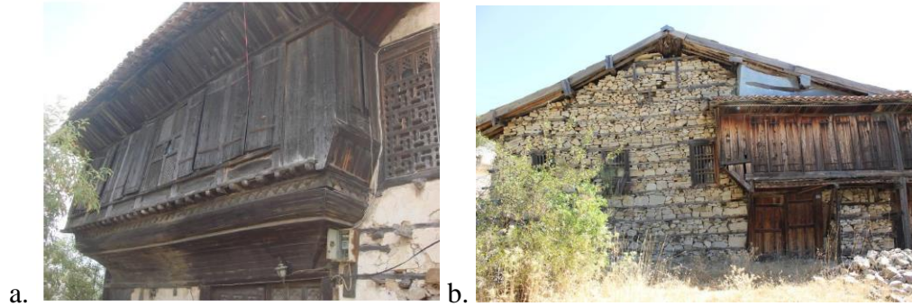
Figure 8a. Example of overhang in Akseki dwelling (Sağiroğlu et al., 2016); 8b. Facade example in Akseki dwelling (Karayazı, 2015)
