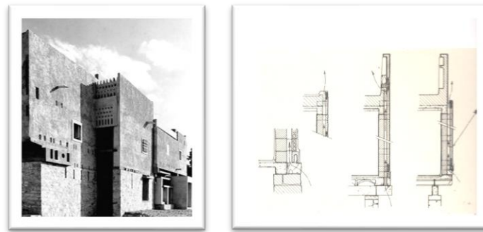
Figure 1. Ghardaia Post Office, The ventilated façade of the case study (Author, 2021).
