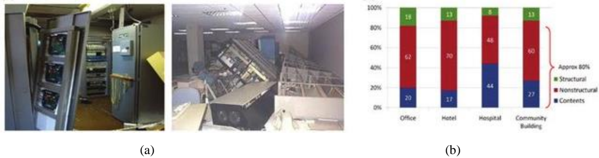
Figure 8. (a) Earthquake damage situations of non-structural components (b) Cost ratio to recover earthquake damage (Sang-Moon Lee & Woo-Young Jung)
