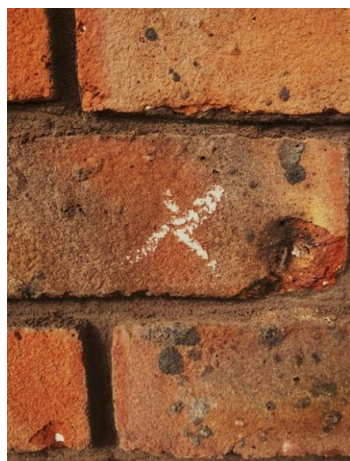
Figure 6. Lime blowing (URL-4)
