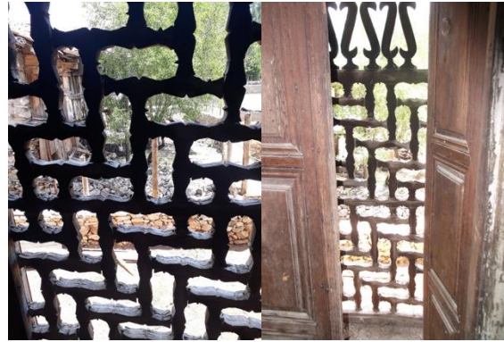
Figure 17. Window with external fence and internal shutter
