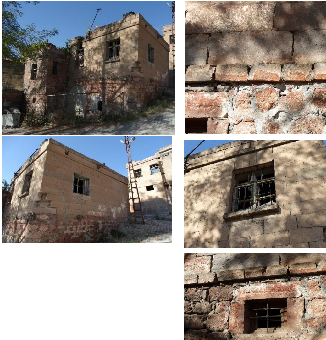
Figure 4. One of the traditional houses in Reşadiye village
