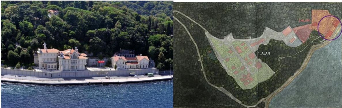
Figure 8. Huber Kiosk General View (Eroğlu, 2012) and Site Plan (Tüfekçi, 2015)
