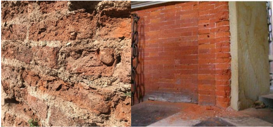
Figure 17. (left). Salts causing exfoliation on the surface (Eryiğit Şenel, 2022)
