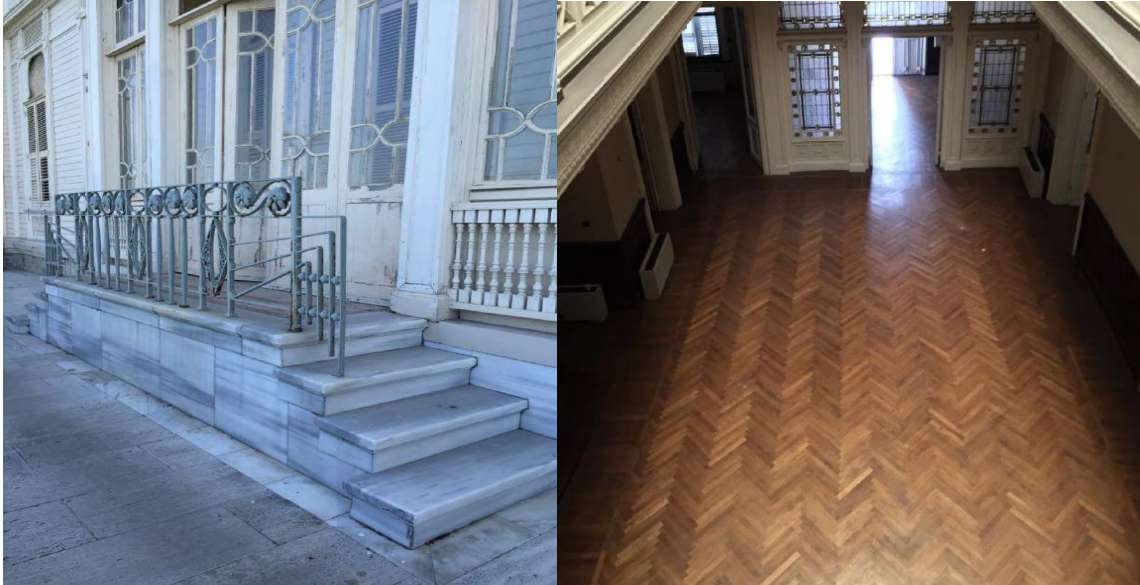
Figure 12. Huber Kiosk Stairs and Interior Pavement (Tüfekçi, 2015)
