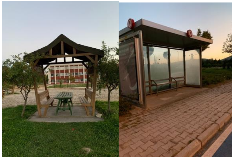
Figure 11. Examples of reinforcement elements in the university
