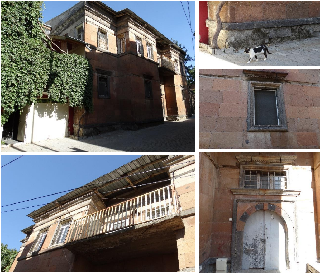
Figure 5. One of the traditional houses in Zincidere village
