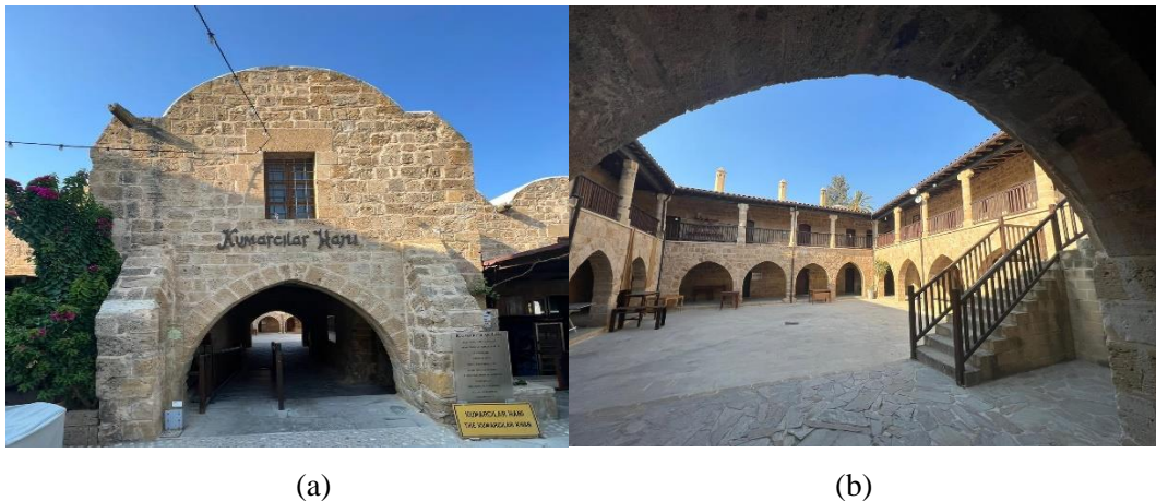
Figure 1. a. b. The Kumarcılar Khan is one of the historic structures built using yellow stone material in the Ottoman period in Cyprus (Öge, 2022).
