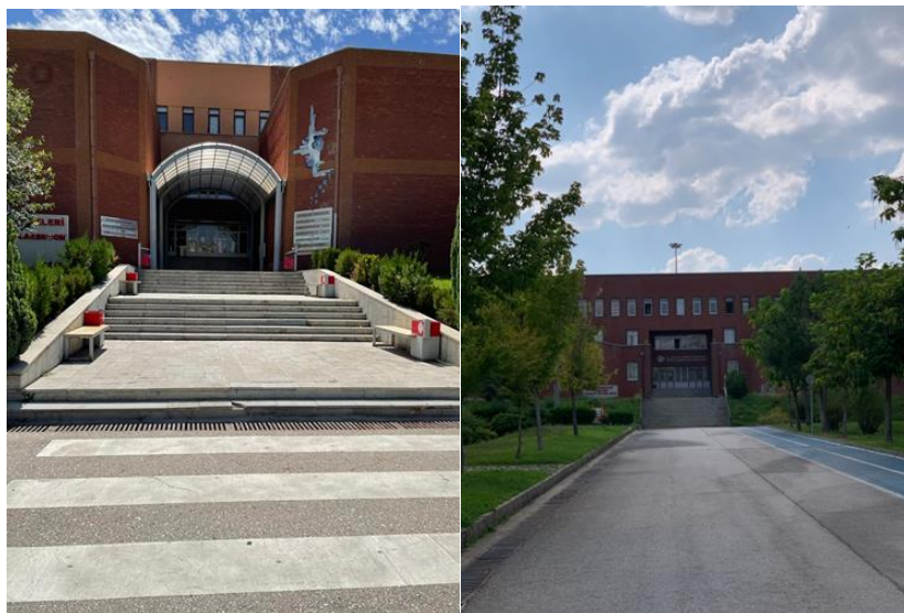
Figure 7. Examples of stairs at university building entrances
